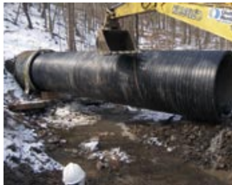
The culvert was sliplined with DN/ID 96 inch (approximately 2.4 m) Weholite. With a small work force of only four men, the team completed the project in record time.
